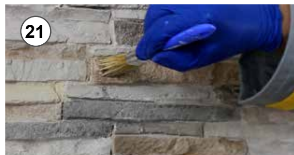
21 - Ossidatura giunto colore marrone 21 - Joint oxidizing by brown colour
