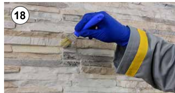
18 - Ossidatura giunto colore beige 18 - Joint oxidizing by beige colour
