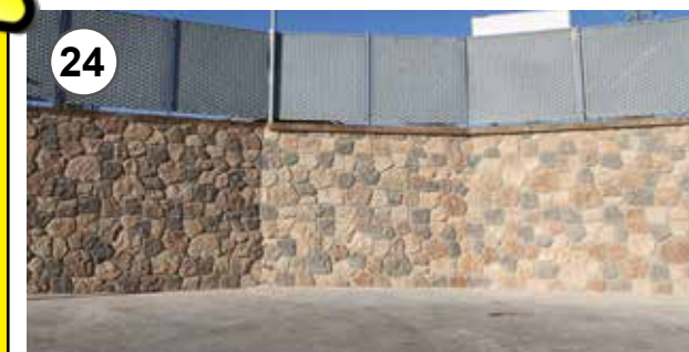
24 - Lavoro ultimato 24 - Completed work
