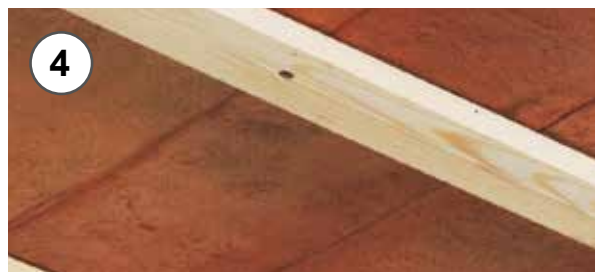
4 - Fissaggio listelli con viti e tasselli 4 - Wooden lath fixing by screws and dowels.
