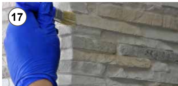
17 - Ossidatura pietra colore beige 17 - Stone oxidizing by beige colour
