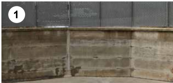
1- Muro grezzo da rivestire 1 - The wall to be covered
