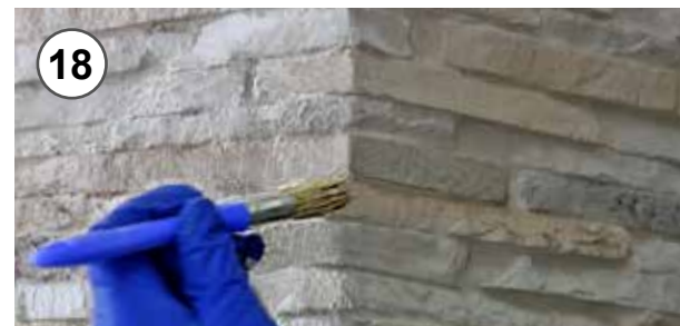
18 - Ossidatura pietra colore giallo 18 - Stone oxidizing by yellow colour
