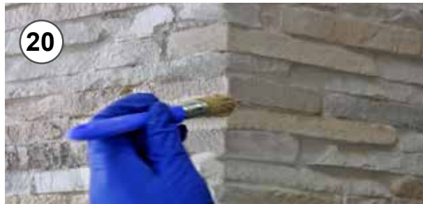
20 - Ossidatura pietra colore marrone 20 - Stone oxidizing by brown colour
